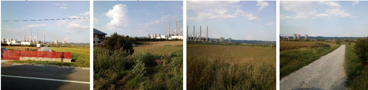
Figure 3: TTPP and the expropriated lands on which the access roads were built and expanded
