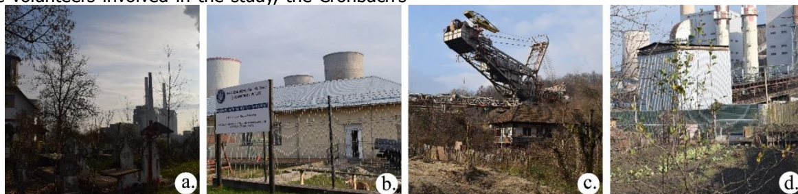
Fig. 2: Aspects of the environmental conflict in the vicinity of the Rovinari thermal power plant are Rogojel Church (a.), Rogojel Kindergarten (b.), house threatened by the presence of a mining machine (c.), and sound-absorbing fences (d.)
