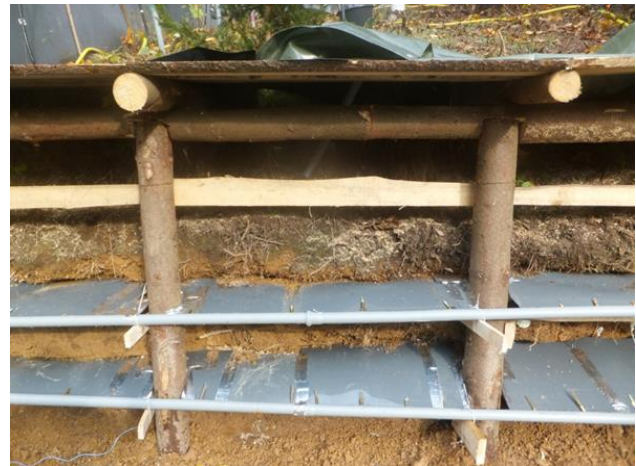
Fig. 2: Troughs (flumes/gutters) in the dug-off slope
